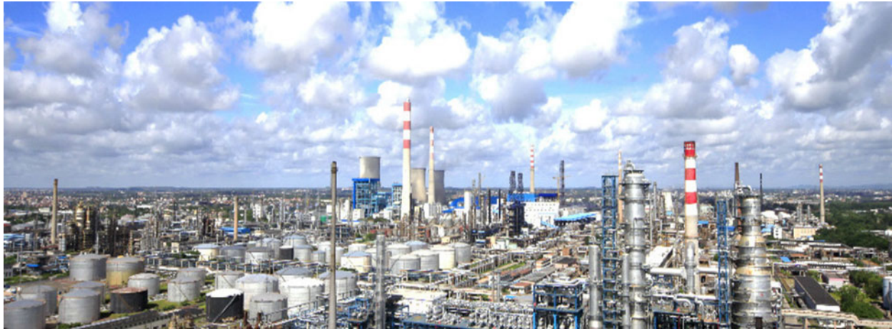
Fig. 1. Example of large-scale petrochemical industry (©SINOPEC Maoming Petrochemical Company (Maoming Company) [Online]: http://www.sinopecgroup.com/group/en/ ) that consists of petrochemical materials, iron and steel pipes, a large variety of equipment, and factory buildings.
